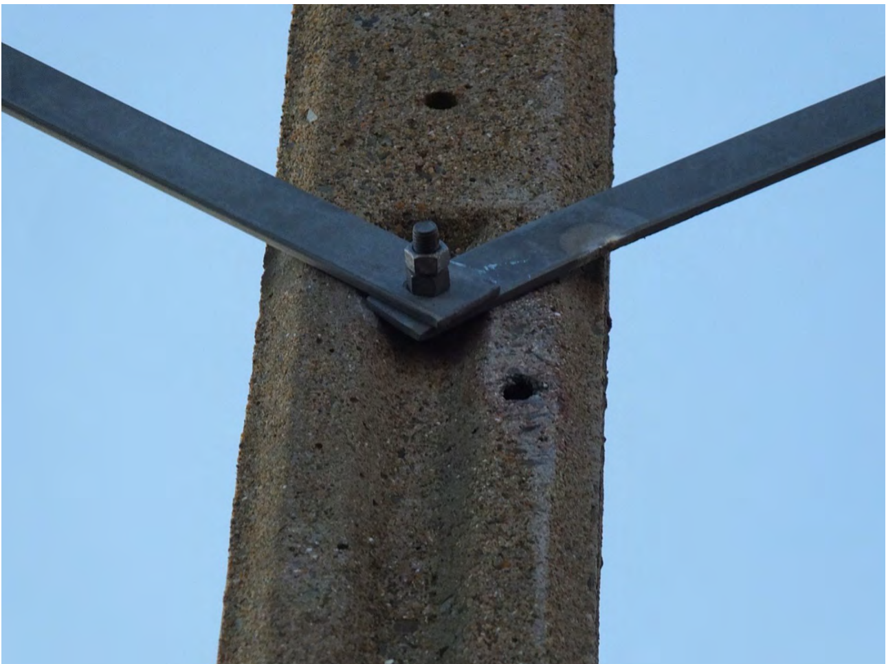
Close up of stay arms on pole 35693 showing the lower arc mark on the right metal stay arm, a hole below the stay arm and what appears to be a scrape mark below this stay arm.
