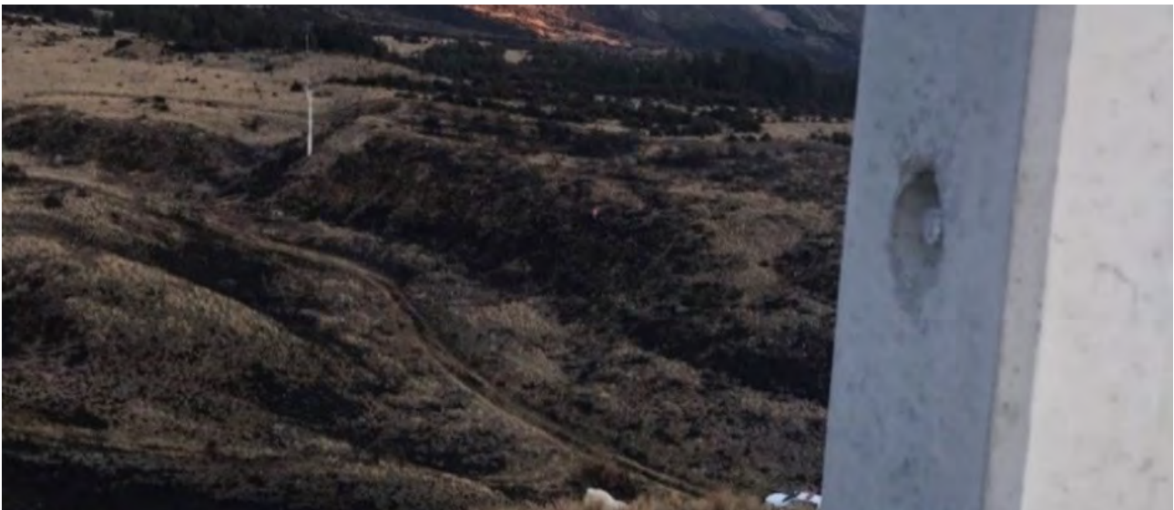
Span from Pole 870452 to Pole 821215 - 175m
