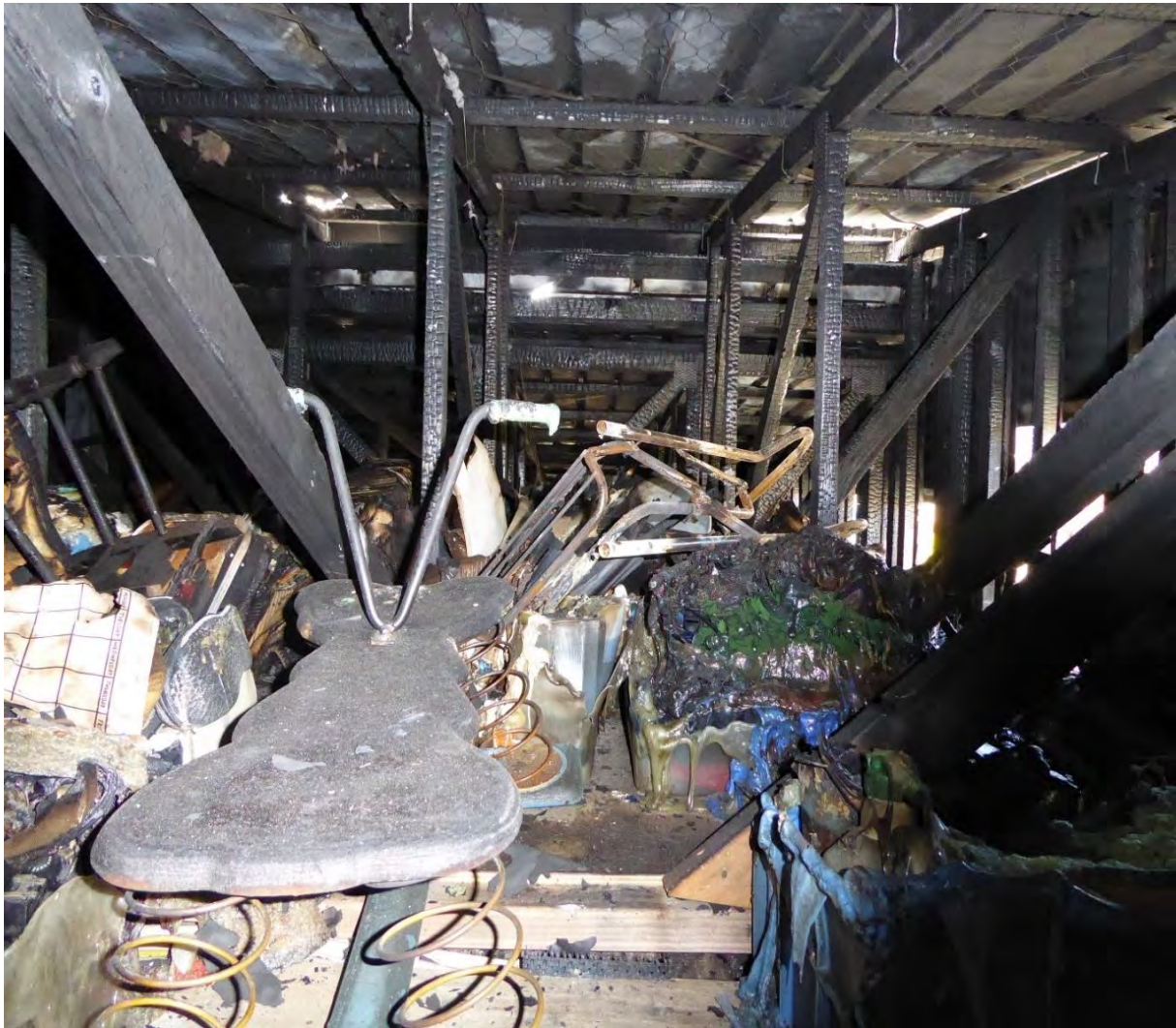
Fig. 18. A crew of firefighters entered this smoke-logged building, accessed the roof void by removing sections of ceiling in the lounge and kitchen and applied water into the roof space. This photo is taken in the roof space.
