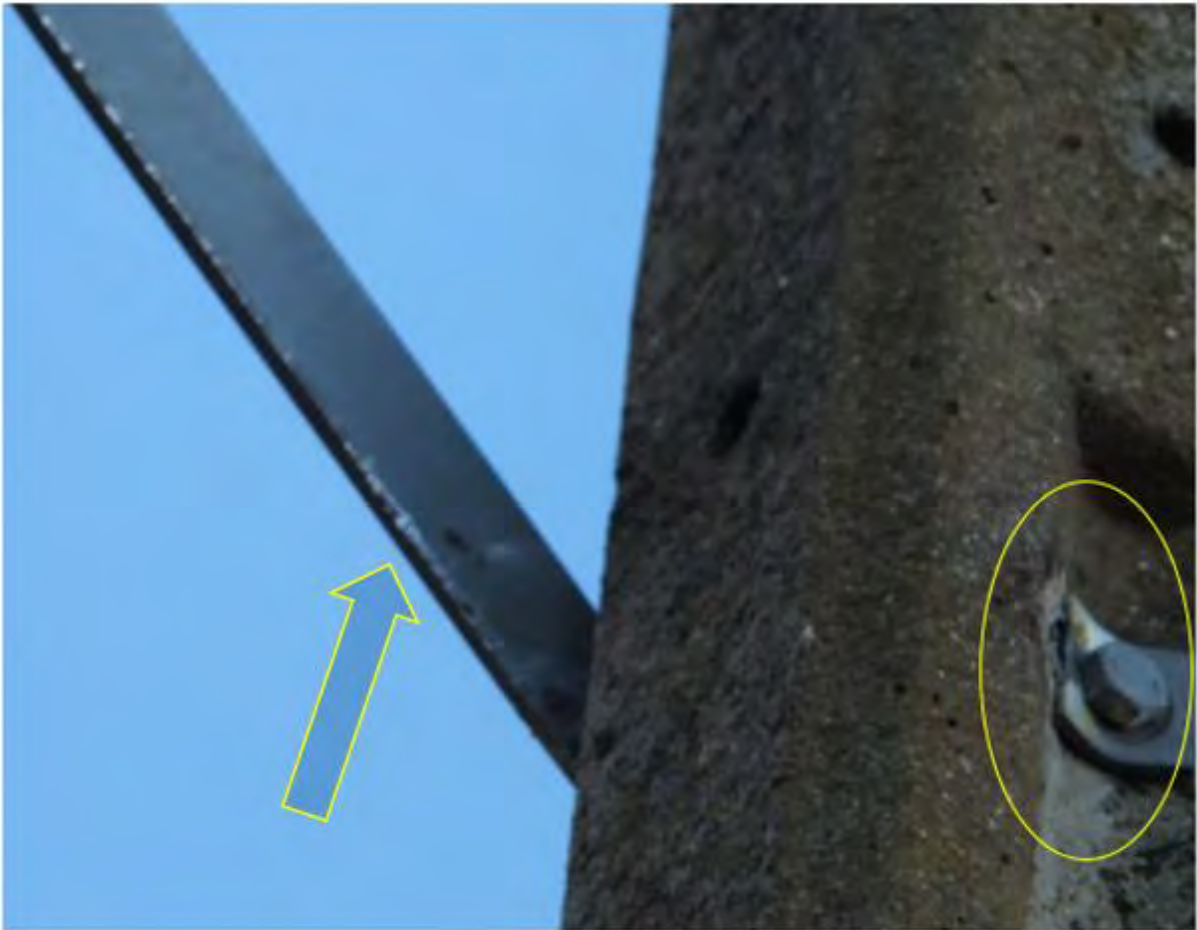
Fig. 49. Photograph (DSCF9369) above identifies location of damage to centre bolt, washer, and damage to edge of metal stay arm.
