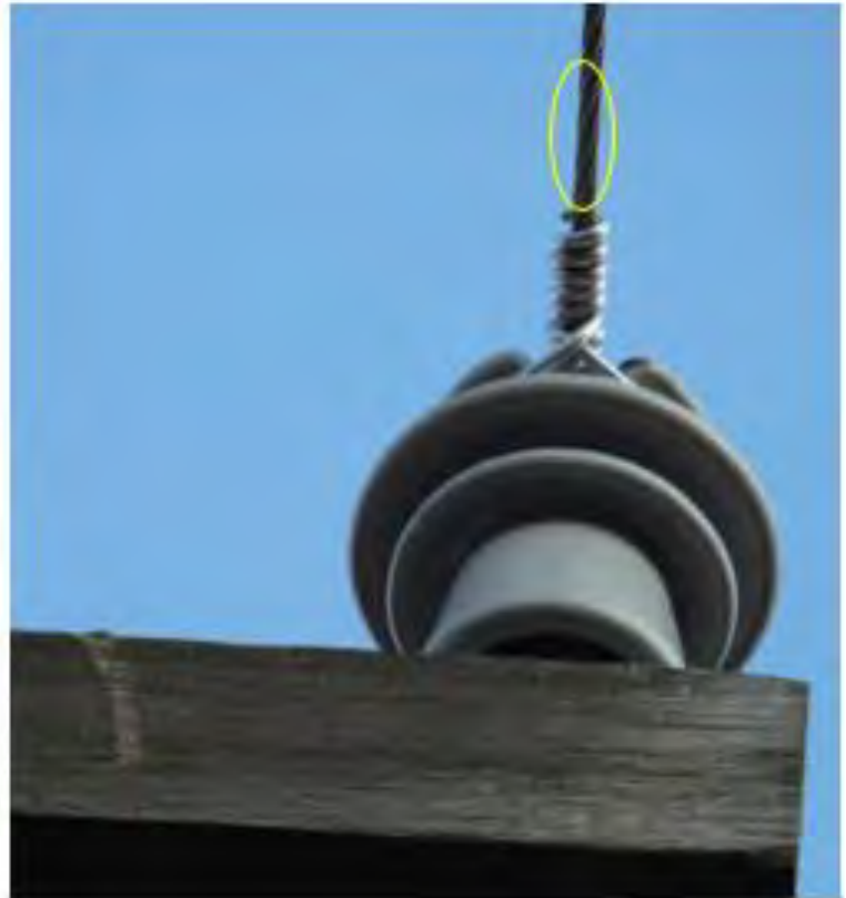
Fig. 51. Photograph above is a zoomed-out image of photograph (DSCF9362) the area within the yellow ellipse shows a rough edge that appears to be damaged.
