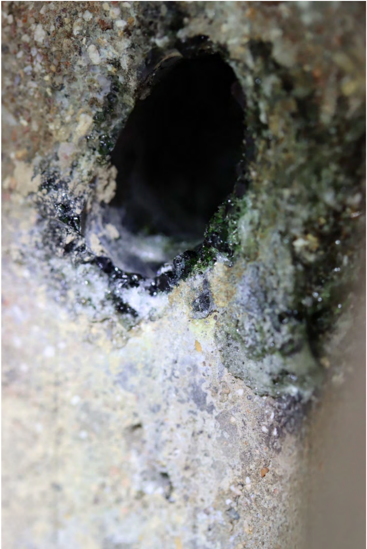
Fig. 72. Burn hole washer side of pole IMG_1452.
