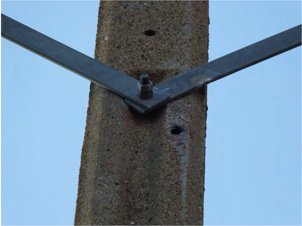
Fig. 48. Photograph (DSCF9365) above shows the lower arc mark on the hillside metal stay arm, a hole below the stay arm and what appears to be a scrape mark on the right-hand side of the pole below the metal stay arm.
