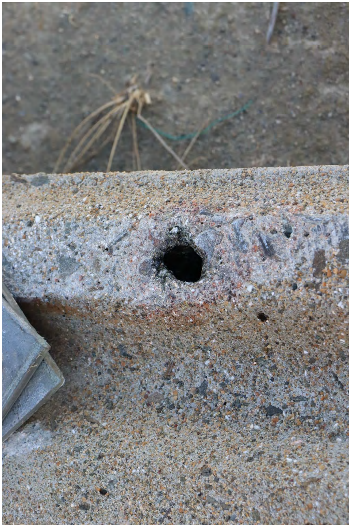
Fig. 65. Close up of the burn hole below the centre bolt holding the metal stay arms to the pole.
