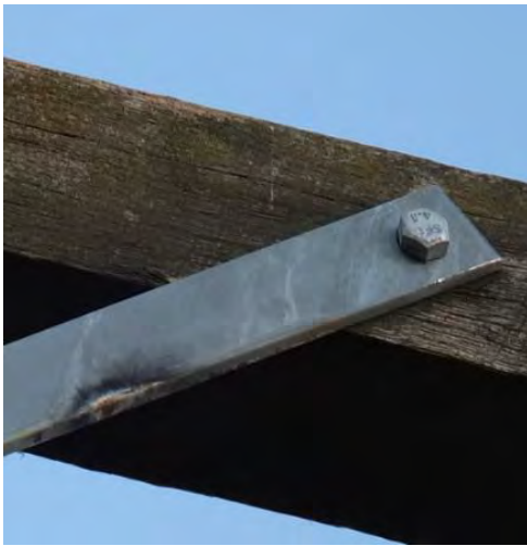
Fig. 45. Photograph (DSCF9361) above left identifies an arc mark to the lakeside metal stay arm on the upper section close to where it is secured to the wooden cross-arm with a double nut.
