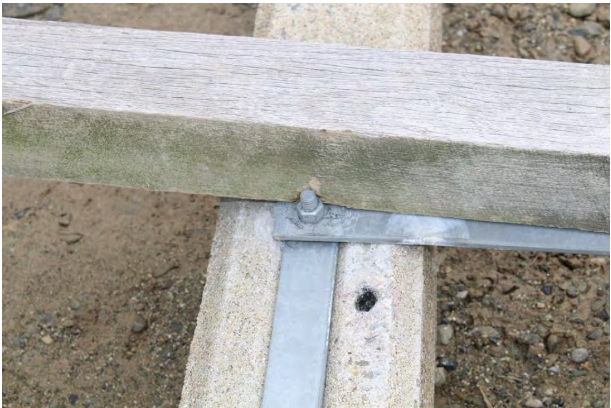
Fig. 60. Close up of cross-arm resting on bolt.
