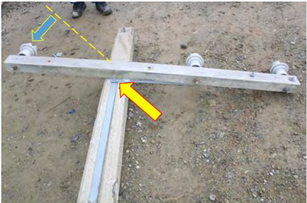
Fig.62. Above, position of metal lakeside stay arm above the RED phase. Held by tension on centre bolt.
