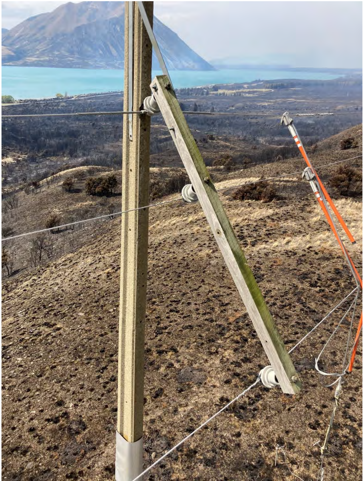
Fig. 55. Photograph (IMG_1711.JPG) above shows the cross-arm rotated over. Photograph supplied by Network Waitaki.
