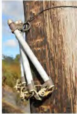
Part Photo DSC\_3367 showing fuse carriers tied to Pole AX728. These do not correspond to those on the Pole at left, as they all have fuse tails in the holders (indicating intact fuses).
