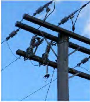
Part P2130031 showing the ruptured fuse tube captured in the White phase fuse carrier and the earth cable clamp. Note appendages on the fuse carrier.
