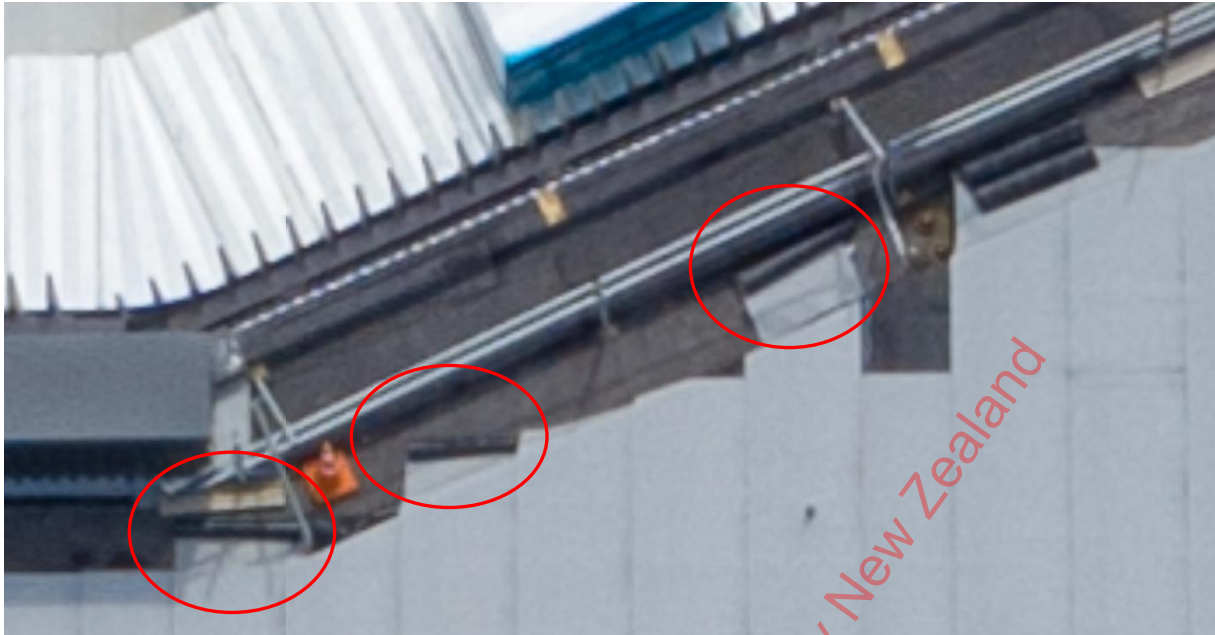
Photo 39: Three examples of residual rolls appearing to be still joined to laid Cap Sheet.
