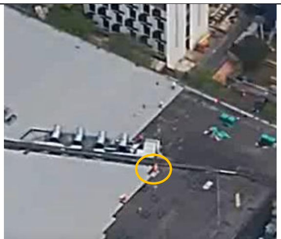
Photo 38: Roofer extends Cap Sheet to gutter while walking behind it. This would exclude the Cap Sheet being an unrolled section which could not be positioned if the worker was standing on it.
