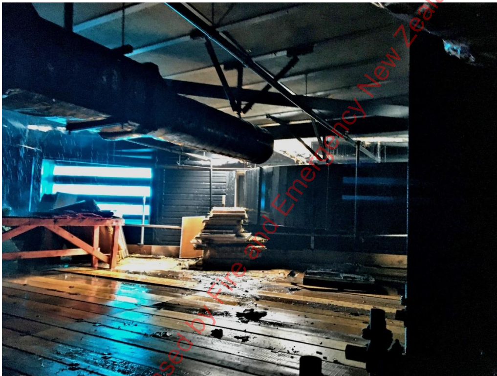
Photo 15: View across the Birds Nest taken approximately 30 minutes after the start of the fire. Visibility was clear and the only fire impact at this stage was from drop down from above. Photo provided by Fletcher Construction.
