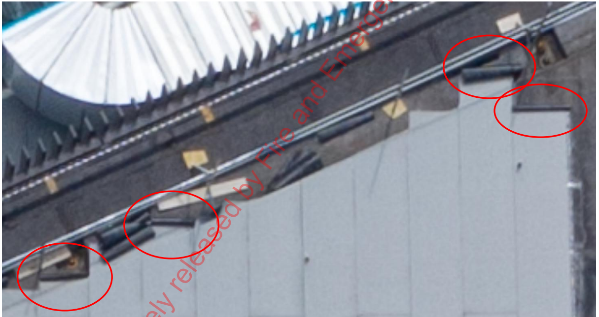
Photo 40: Four examples of residual rolls appearing to be still joined to laid Cap Sheet.
