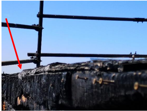
Photo 41: Example of roof on western side of Level 7 near the area of origin with top plywood sheets overlapping vertical plywood.
