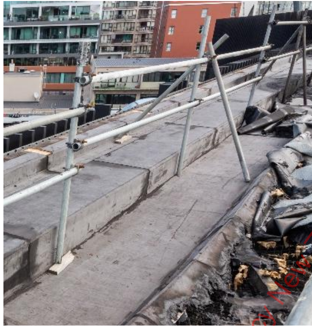
Photo 25: Example of guttering on eastern side of Level 7 with Base Sheet complete.
