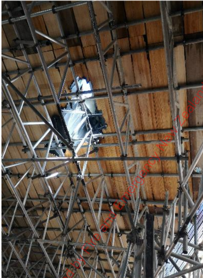
Photo 16: Burn damage to 'Birds Nest' floor caused from burning debris dropping from above the scaffolding floor.
