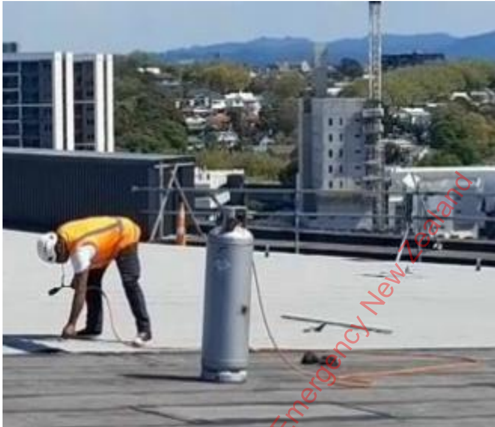
Photo 45: Shows an un-tensioned gas hose falling slack beside A gas cylinder and slack in the hose on the ground. Photo provided by Worksafe.
