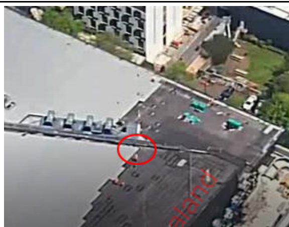
Photo 34: Shows Cap Sheet complete to gutter edge at 12:20 p.m.
