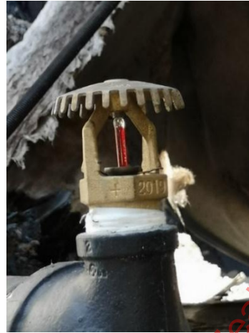
Photo 17: Example of a quick response sprinkler head under the ceiling in the area of origin with bulb still intact.
