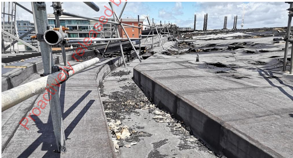
Photo 20: Shows a comparable view of the gutter on the east side of the Level 7 roof after the fire showing the Base Sheet installed. The Cap Sheet had not been applied in this location.
