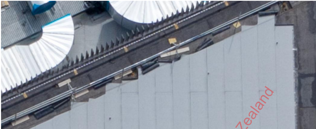
Photo 21: A photo taken 2 days before the fire shows the Cap Sheets laid to the edge of the gutter and residual rolls left lying in the gutter area. Photo supplied by Fletcher Construction.
