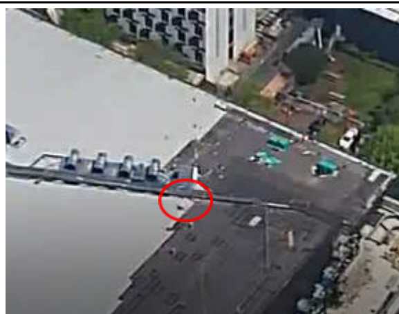
Photo 33: Shows Cap Sheet at 12:17 p.m. incomplete to gutter edge.
