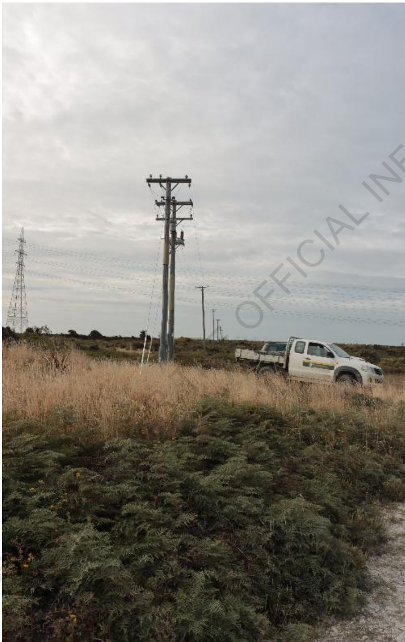
Photo 3: 11kv distribution line.
