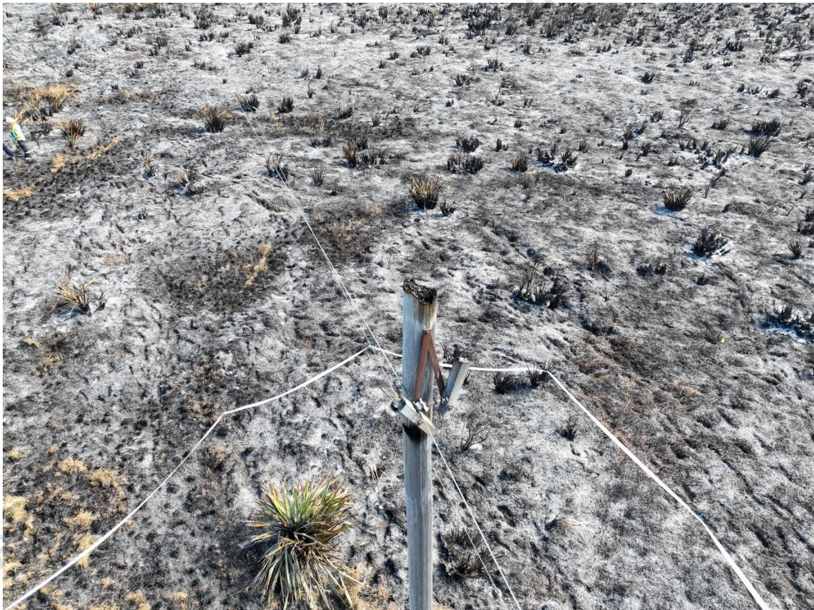
Photo 4: Fire damage to top of pole 6 and the crossarm.
