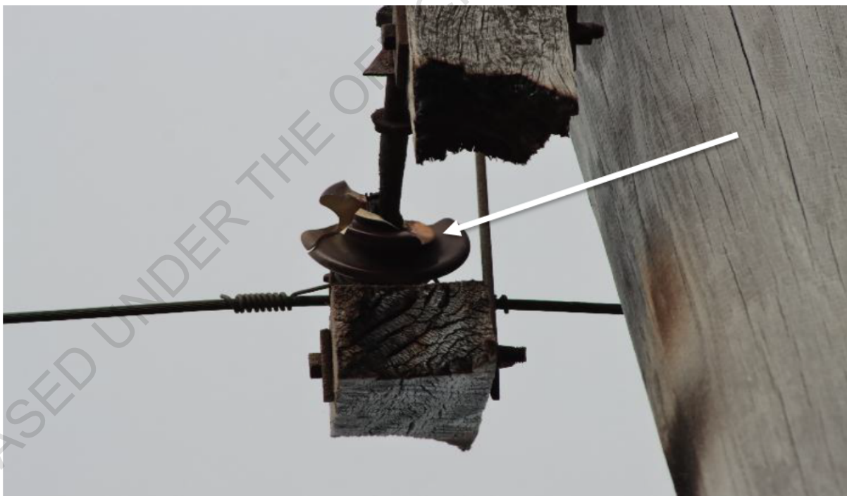
Photo 14: White arrow indicates a damaged insulator still on the powerline. Damaged insulator resulted in a phase to earth fault.
