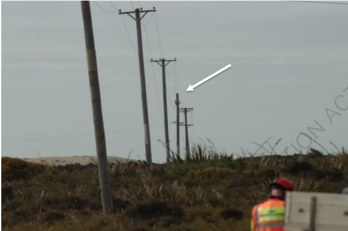
Photo 11: Distribution line to NZAS bores. White arrow indicates damaged pole 6.
