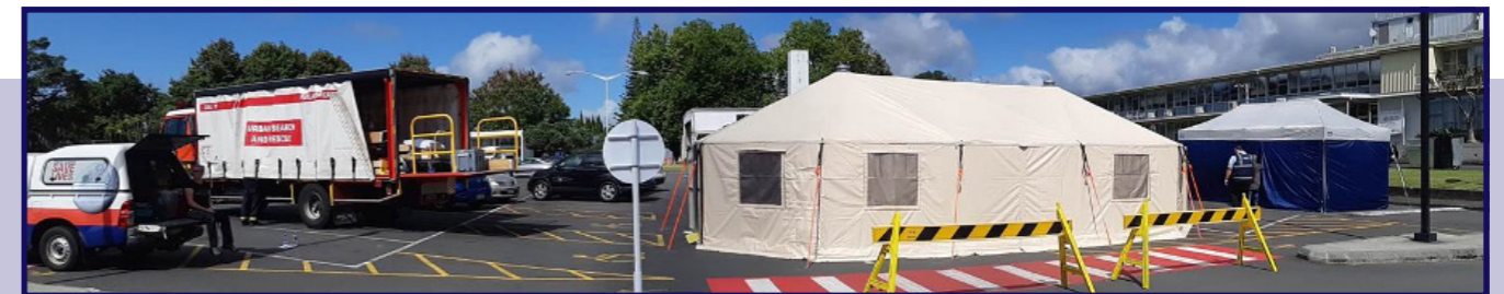
Construction of the screening facilities outside Waitakere Hospital
