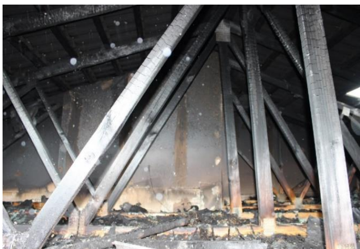
Image above shows fire damage in ceiling space of fire affected unit. The fire separation wall is visible in the rear of image.
