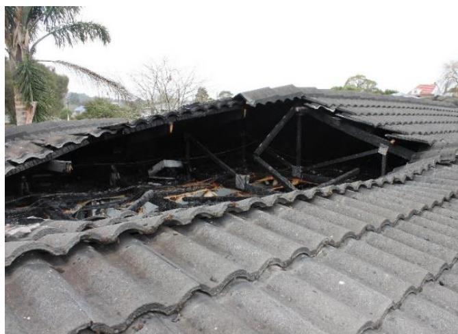
Image above shows partial roof collapse on the fire side of the separation wall.
