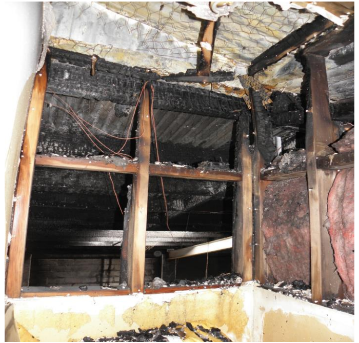
Figure 2 - First Incident: remnants of the wall separating the kitchen of the residential unit from the workshop
