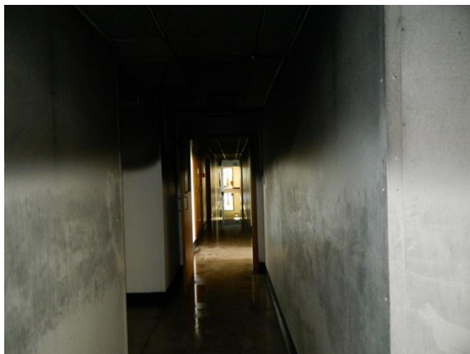
Figure 2: Showing extensive smoke damage throughout building
