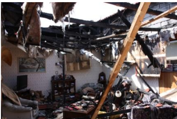
Photos showing damage in adjacent units as a result of fire spread.
