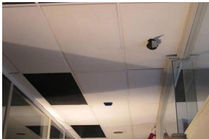
Fluorescent light units and other openings allowing smoke travel.
