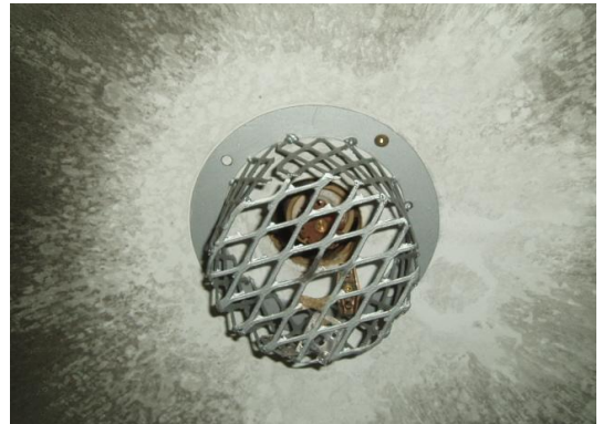
Guard fitted to sprinkler head in room of fire origin
