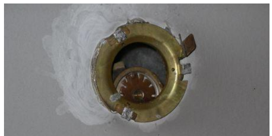
Recessed sprinkler head in hallway unable to drop down
