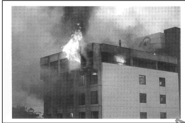
Figure 2.24: Flames from the window indicate a ventilation-controlled, post-flashover fire (Source: Fire Engineering Design Guide – Buchanan)
