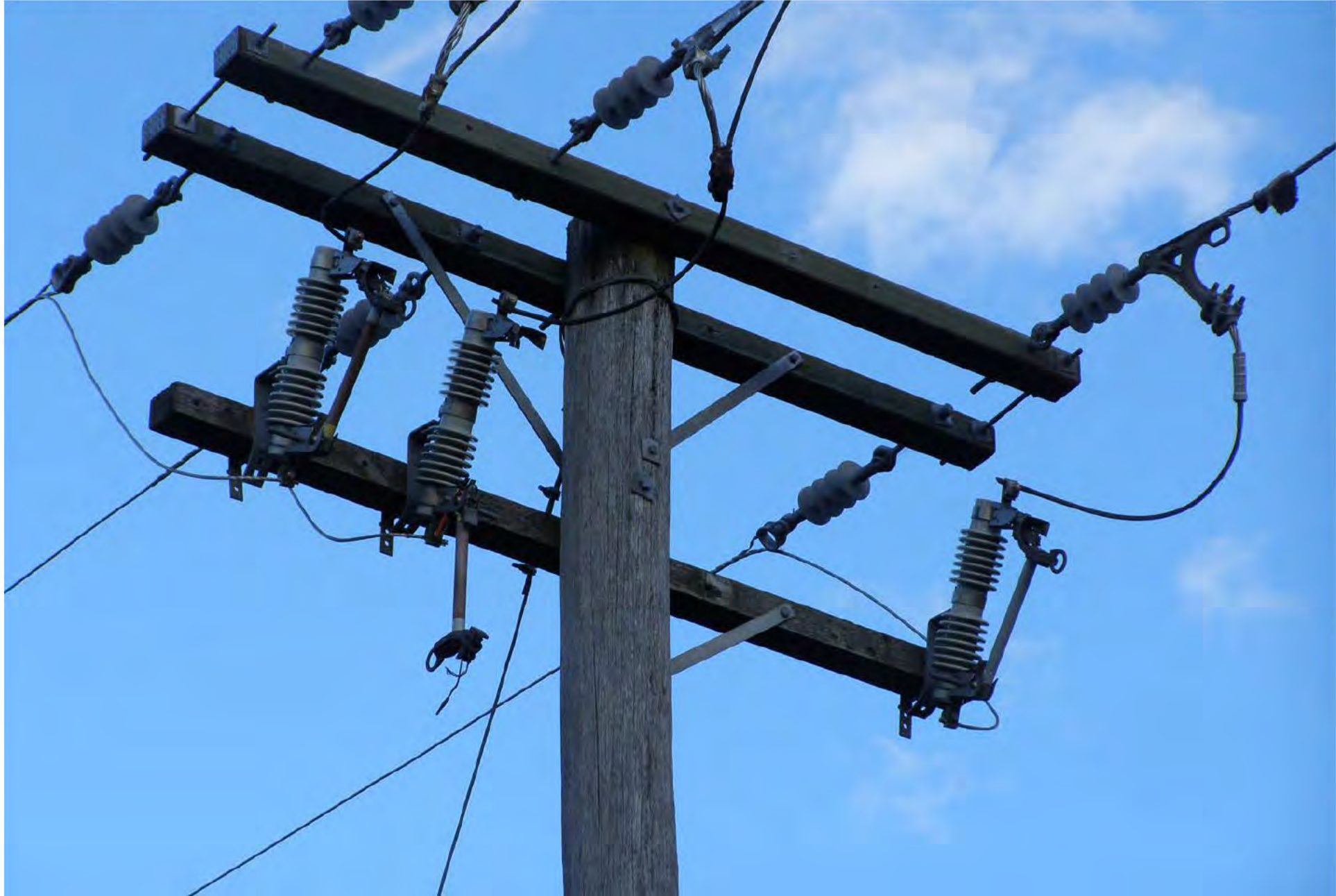
Photo 2130031–Pole AX728, shows ruptured fuse. Note appendages hanging from fuse carrier and remains of fuse tube (orange) held in earth clamp
