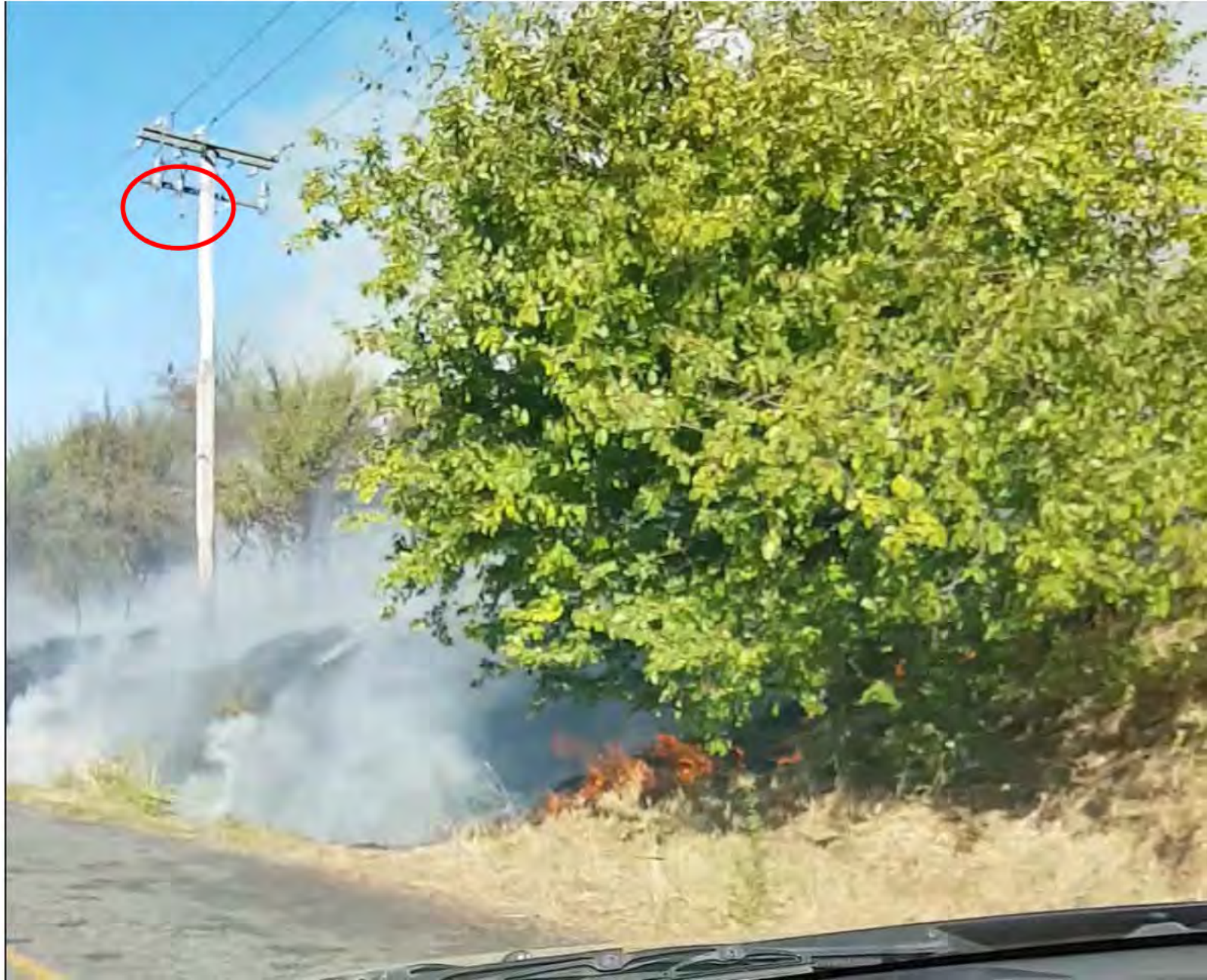
IMG OMG9 – Fire location reference image of Pole AX728 taken from OMG video at 17:51 (note fuse has ruptured)
