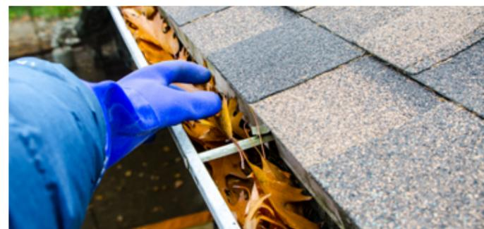
Figure 10: Example of debris accumulation in gutter
