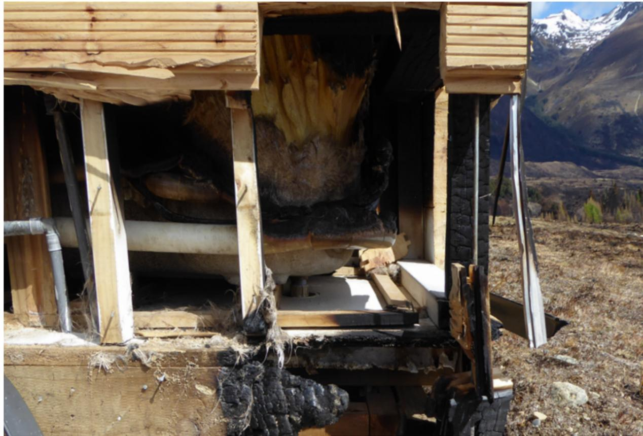
Figure 12: Example of how vulnerable timber cladding is to ember attack, radiant heat or direct flame. Fire has broken through and set bathroom inside alight. Ōhau 2021 (Fire 3088958)
