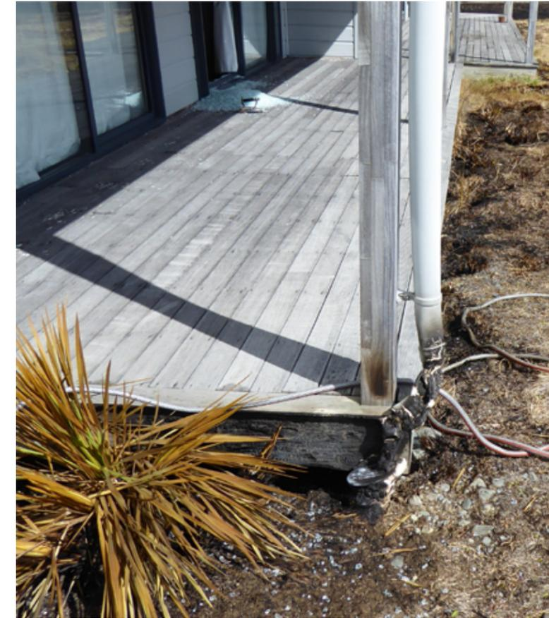
Figure 17: Example of how vulnerable wooden decks are to being ignited via direct flame, ember attack or radiant heat exposure
