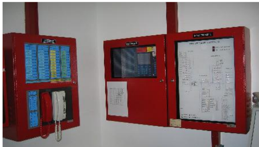
Figure 6 – Some of the equipment found in a typical FCC
