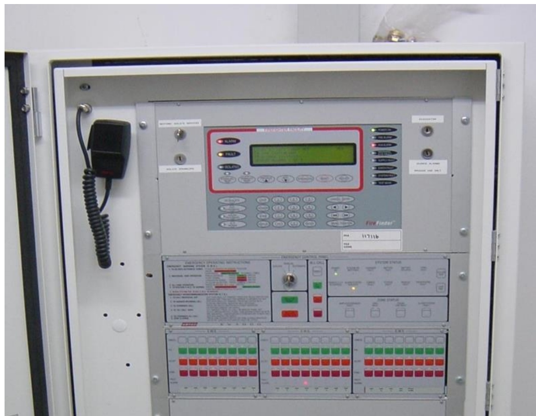
Figure 8 – EWIS panel with analogue addressable display
