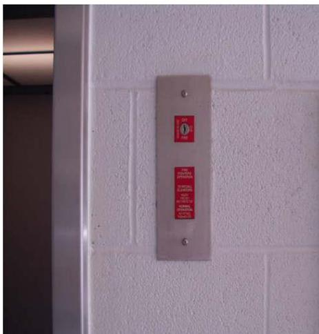
Figure 3: Designated recall level showing the lift key location
