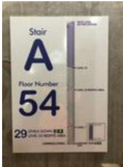
Figure 2 – Example of stair signage
