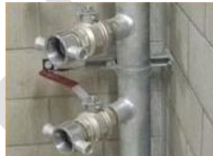
Figure 5: Typical charged riser outlet
