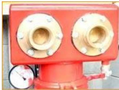
Figure 4: Two-way charged riser inlet
