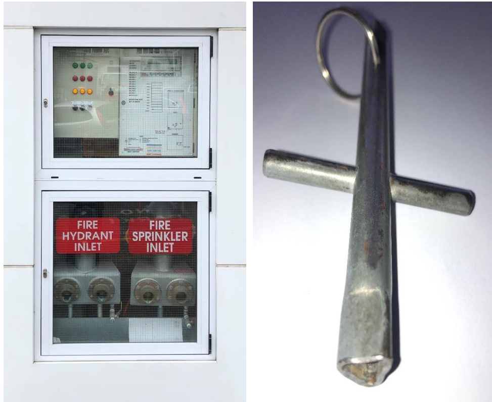
Figure 6 – Glass-fronted enclosure with triangular key access and a triangular key
