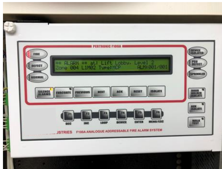
Figure 2 – Functions of an analogue addressable system
