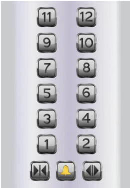
Figure 2 – Lift floor numbering which replicates the fire alarm panel floor numbering
