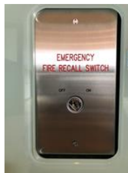
Figure 1 – Firefighter control recall switch
