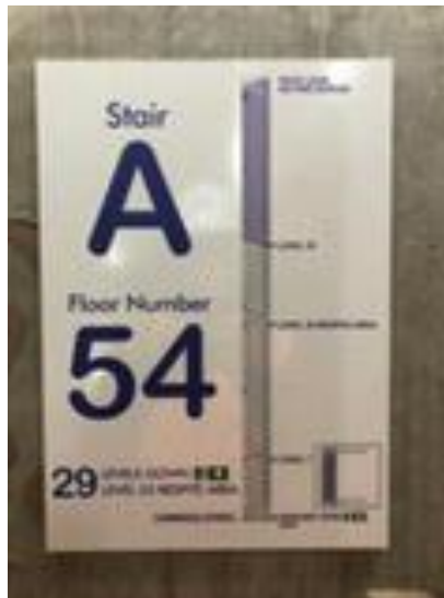
Figure 2 – Example of stair signage
