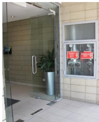
Figure 9 – Hydrant inlet located creating trip hazard
