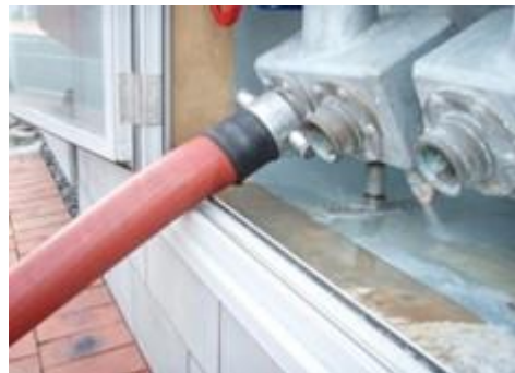
Figure 6 – Insufficient clearance, hose rubs on bottom edge
