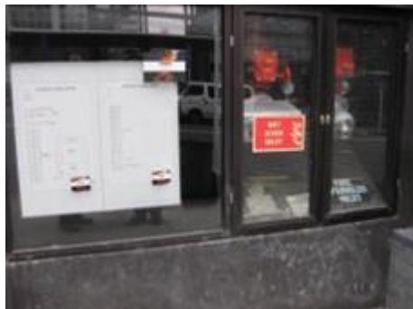
Figure 5 – Clear space, sloping splash guard to base
