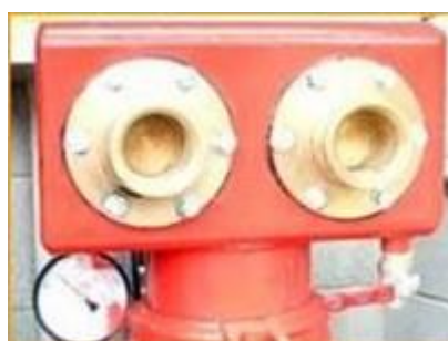
Figure 2 – Two-way charged riser inlet
