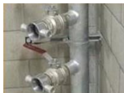
Figure 3 – Typical charged riser outlet
