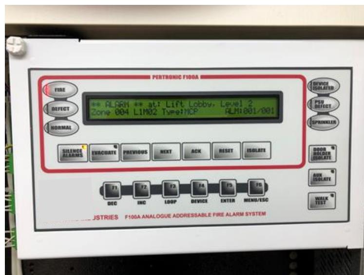
Figure 2 – Functions of an analogue addressable system
