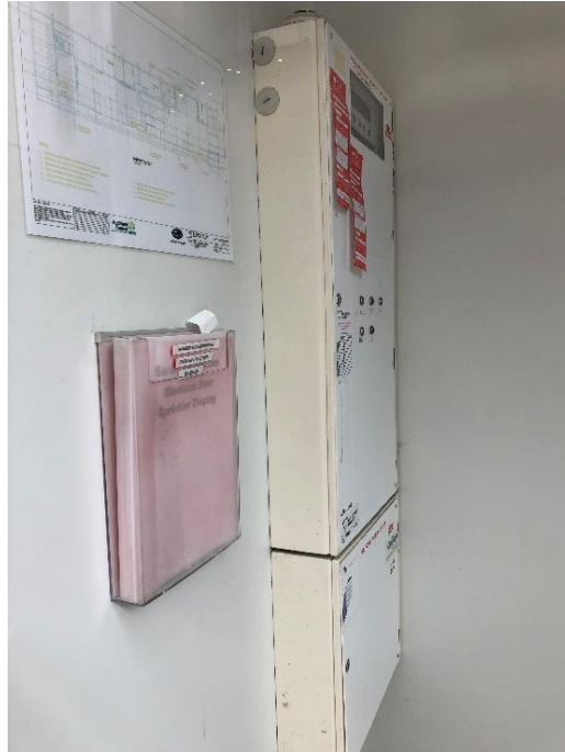
Figure 8 – Hard copy information and diagrams clearly located with the main panel
