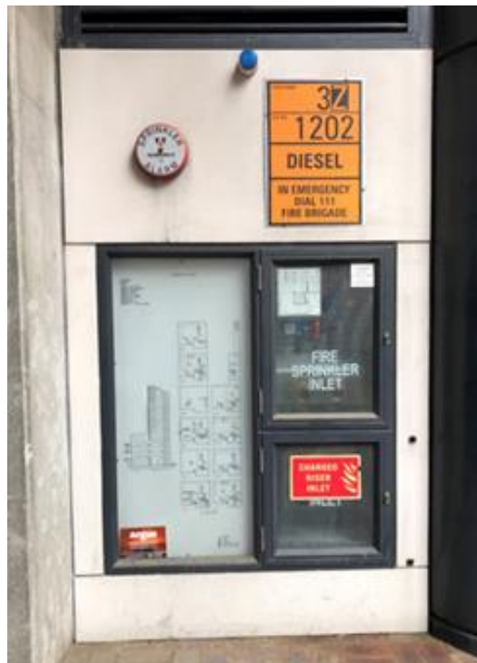
Figure 3 – Panel co-located and identified with a blue strobe
